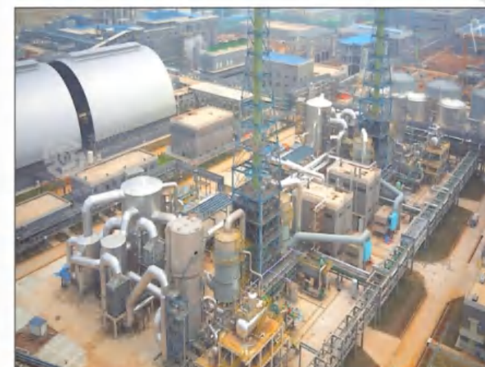
Henan Branch Bangpu Yihua Supporting Raw Materials and Iron Phosphate Engineering Project
