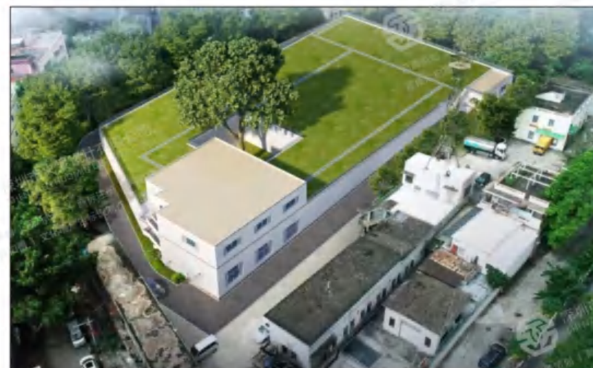
Guangzhou Water Supply Company's Permanent Power Supply Project - Huangpu Pressure Station Clean Water Tank Construction Project
