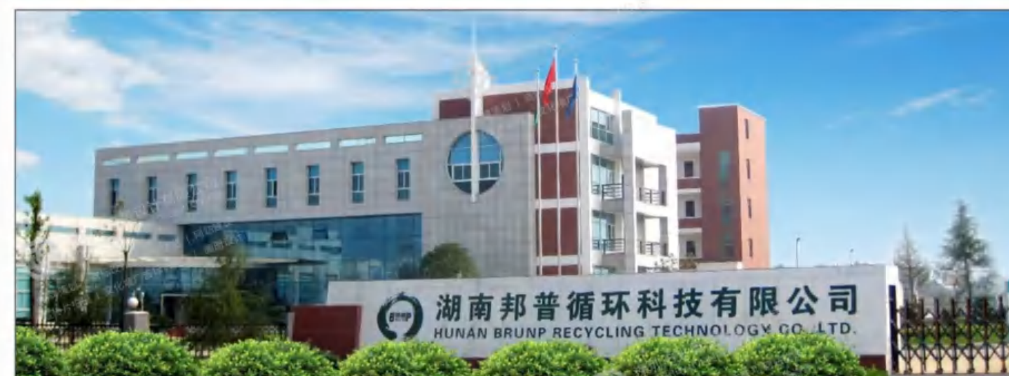
Hunan Bangpu Recycling Technology Co., Ltd. Project
