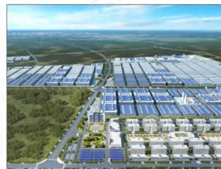
Bangpu Integrated New Energy Industrial Park- Bangpu Era Lithium ion Battery New Materials Project
